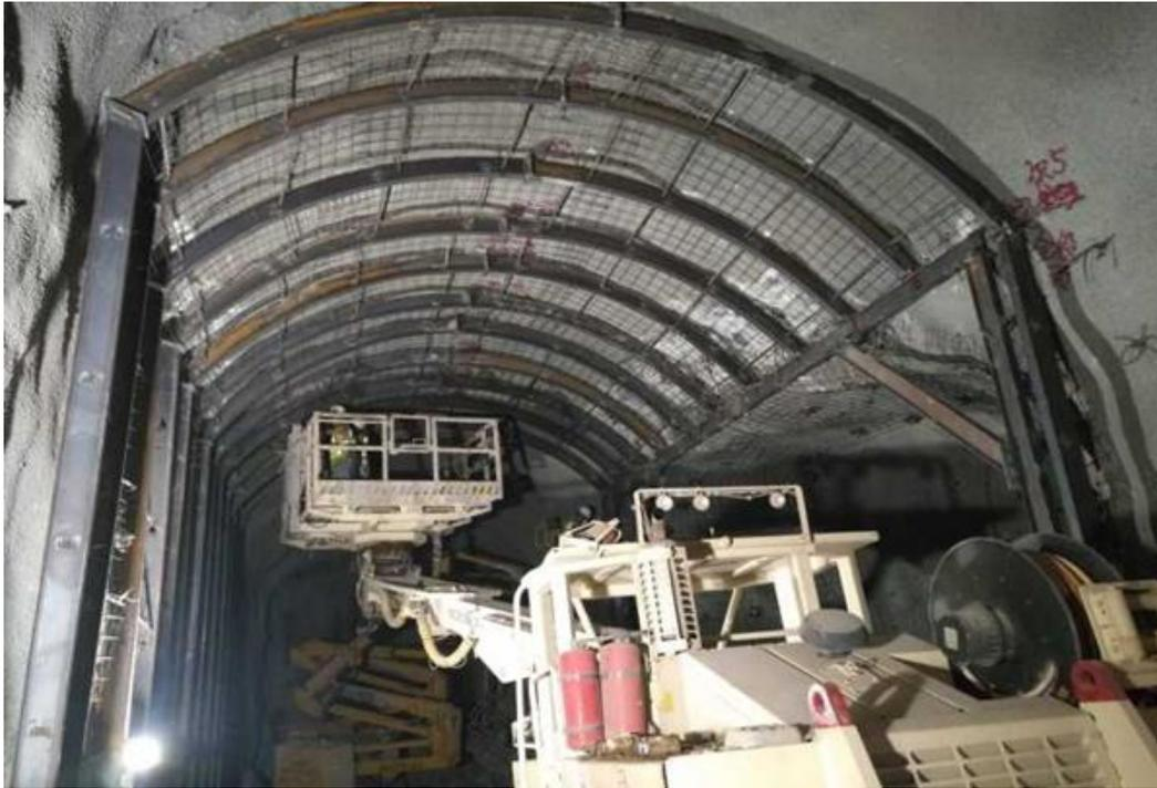
The construction of the #4 Emergency Gallery approximately 1.5km underground from the tailrace access near to the powerhouse cavern location. This is in an area of weak rock geology therefore extensive steel support of the tunnel works is required as shown. The geology is weathered basalt rock.
