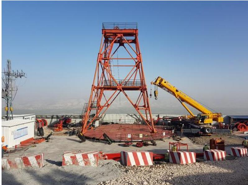
Drilling equipment above the excavated surge shaft. The construction of the 500m vertical pressure penstock (3.5m diameter) will be by the shaft sinking method with material brought to the surface. The design and construction of the shaft is very complex.
