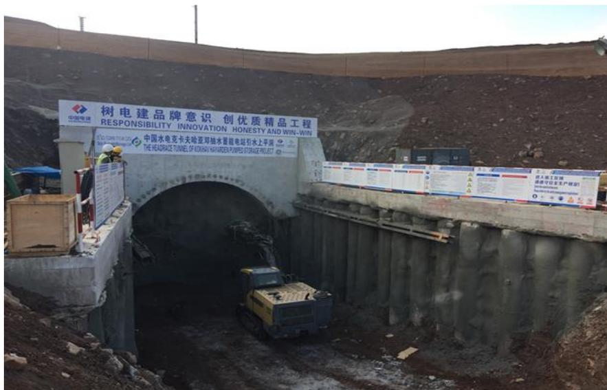
The portal of the upper intake headrace tunnel under construction within the upper reservoir pond
