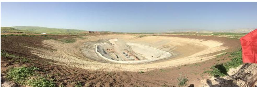
Commencement of the lower reservoir (3MCM) construction to allow the tailrace tunnel portal construction. The pond will eventually become kidney shaped and significantly larger than as shown in this photo.
