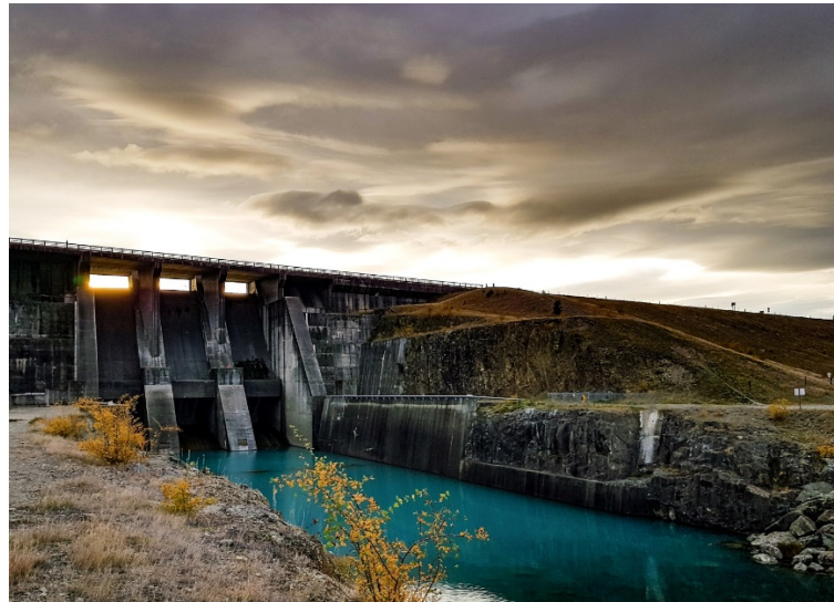
2018 Runner-up: Nicola Ponsonby Ruataniwha Dam and Spillway
