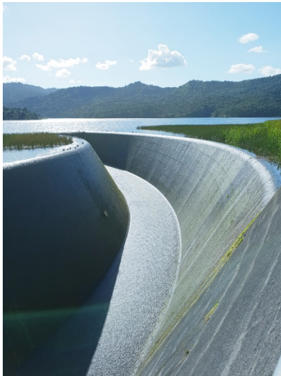
2018 Winner: Kerry Swanepeel Lower Nihotupu Dam Spillway
