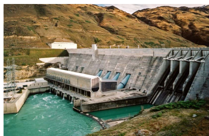
Figure 2. Clyde Dam (the largest concrete gravity dam in NZ) incorporates a slip joint, designed to accommodate up to 2m of movement on the river channel fault [4]
