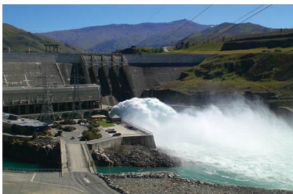
Figure 6.21: Low Level Outlet Structure – Clyde Dam (provided by Contact Energy)
