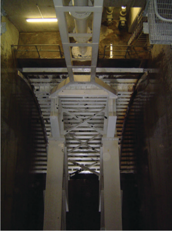
Figure 6.13: Orifice Radial Gate – Clyde Dam (provided by Contact Energy)
