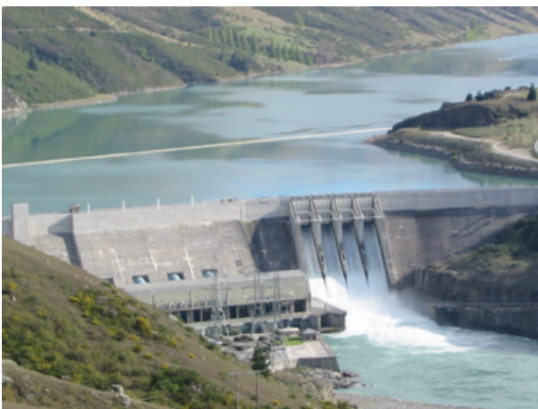
Figure 6.5: Concrete Gravity Dam – Clyde Dam (provided by Contact Energy)
