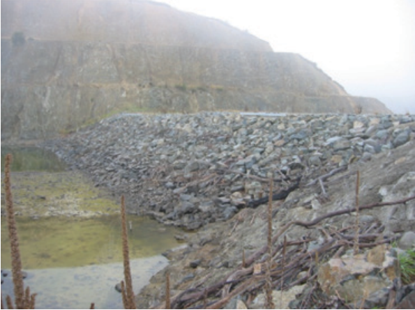
Figure 6.20: Auxiliary Spillway – Opuha Dam (provided by Opuha Water)
