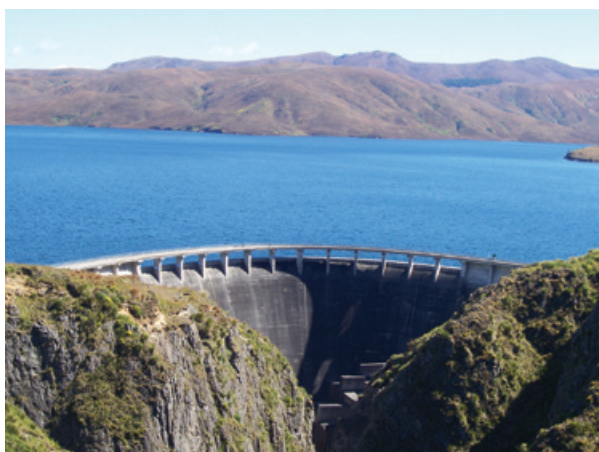
Figure 6.9: Concrete Arch Dam – Moawhango Dam (provided by Genesis Energy)
