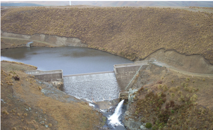
Figure 6.6: RCC dam – Horseshoe Bend Dam (provided by Pioneer Generation)
