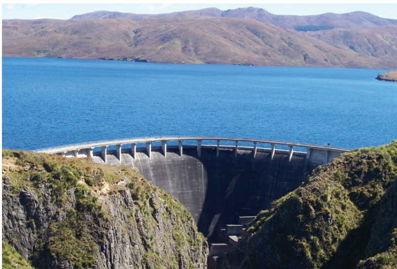
Figure 6.9: Concrete Arch Dam – Moawhango Dam (provided by Genesis Energy)
