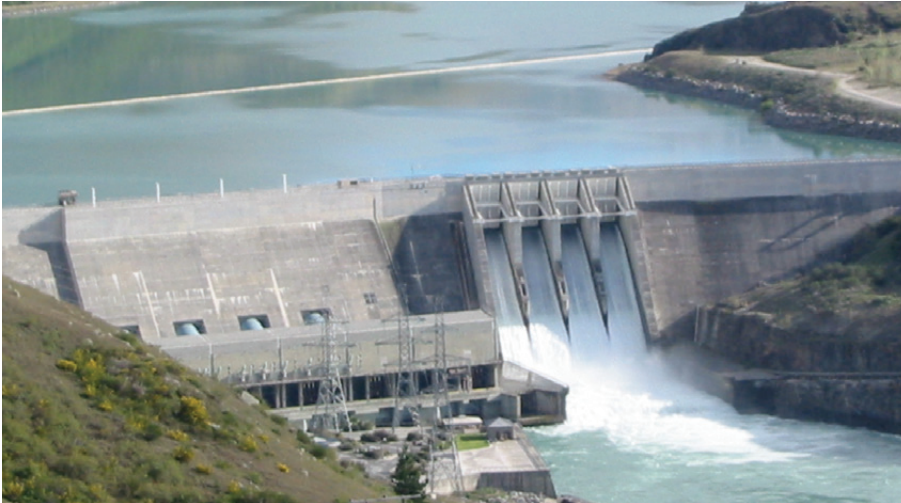
Figure 6.5: Concrete gravity dam – Clyde Dam (provided by Contact Energy)
