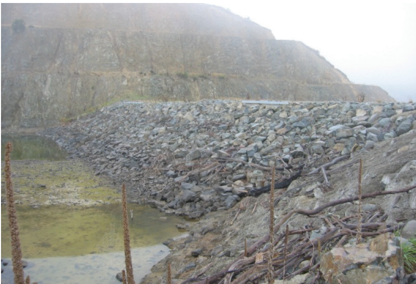
Figure 6.21: Controlled - spillway - auxiliary spill outlet with fusible weir Opuha Dam (provided by Opuha Water)
