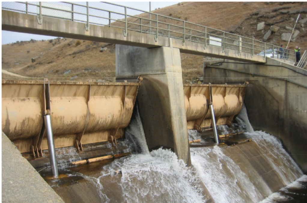
Figure 6.17: Controlled - spill gates - flap gate at Paerau Weir (provided by Manawa Energy)
