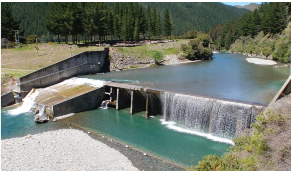
Figure 6.8: Concrete buttress dam – Branch Dam (provided by Manawa Energy)
