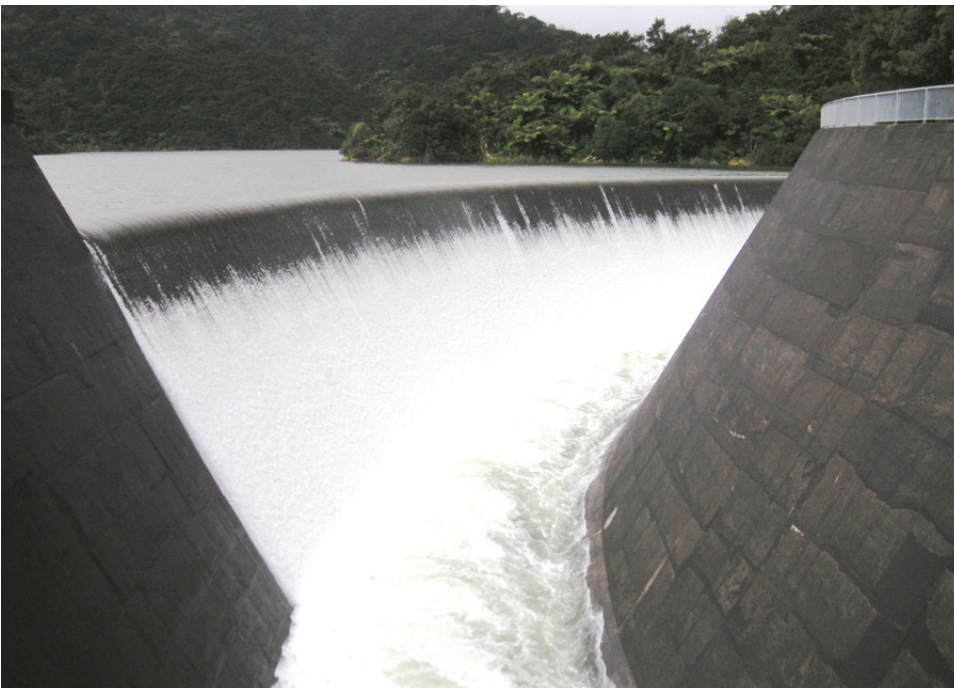
Figure 6.15: Uncontrolled – spillway - lateral or side channel spill outlet – Upper Mangatawhiri Dam (provided by Watercare Services)
