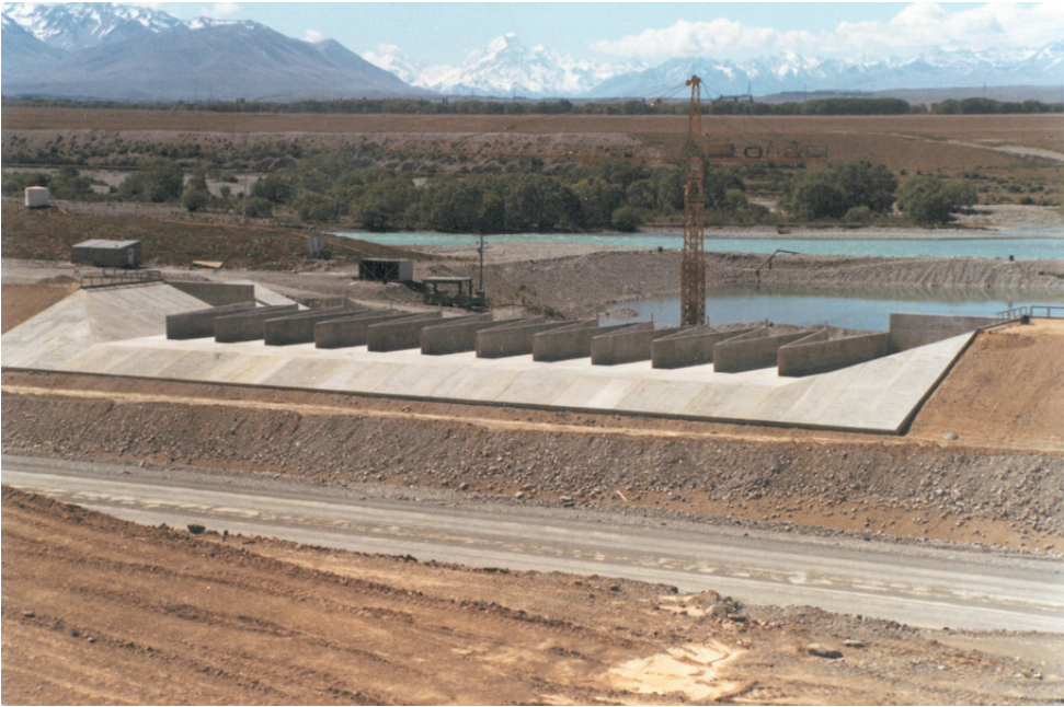
Figure 6.14: Uncontrolled - spillway - side spill labyrinth weir – Ohau C Canal (provided by Meridian Energy)
