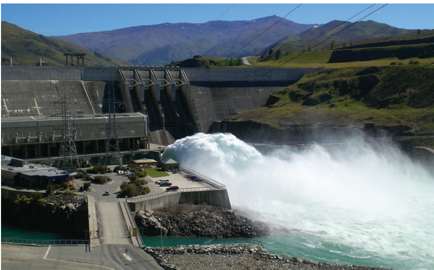
Figure 6.11: Controlled - low-level outlet – Clyde Dam (provided by Contact Energy)
