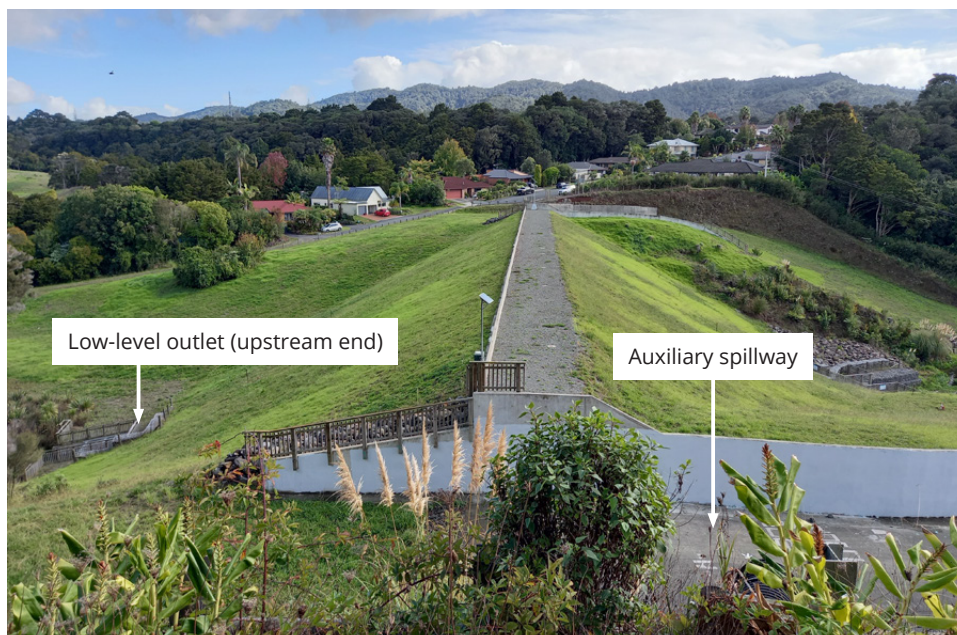
Figure 6.11: Hopua Te Nihotetea flood detention dam on Raumanga Stream, Whangarei, operated by Northland Regional Council (photo provided by Damwatch Engineering)
