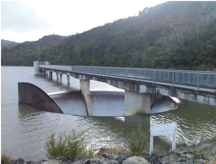
Figure 6.12: Uncontrolled - spillway morning glory spill outlet – Lower Huia Dam (provided by Watercare Services)
