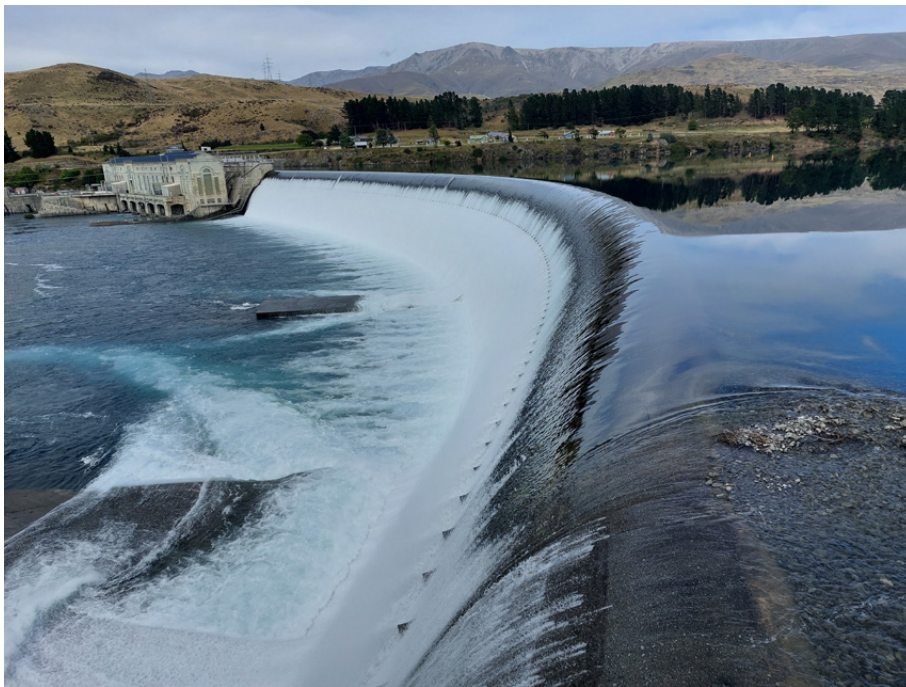
Figure 6.13: Uncontrolled - spillway - free overflow ogee crest weir – Waitaki Dam (provided by Meridian Energy)
