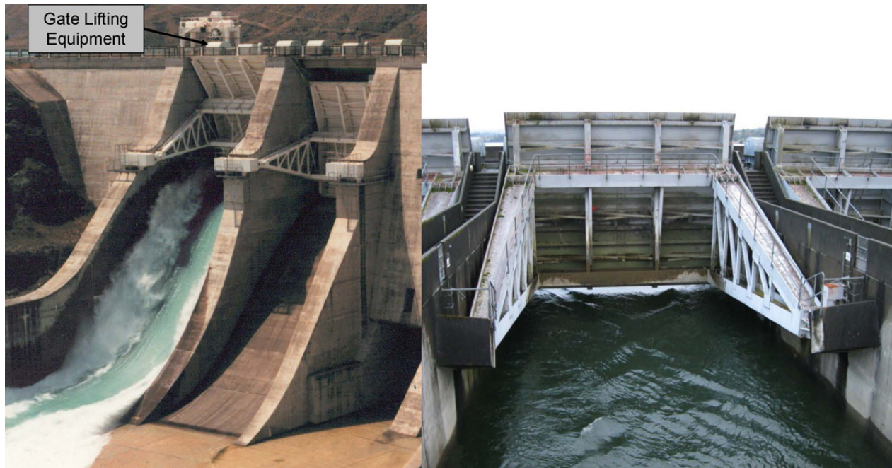
Figure 6.16: Controlled - spillway - radial gate – Benmore Dam & Te Anau Lake Control (provided by Meridian Energy)
