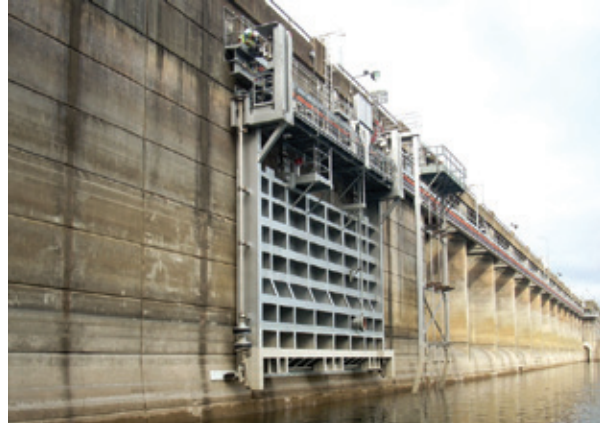
Figure 6.17: Upstream Bulkhead
