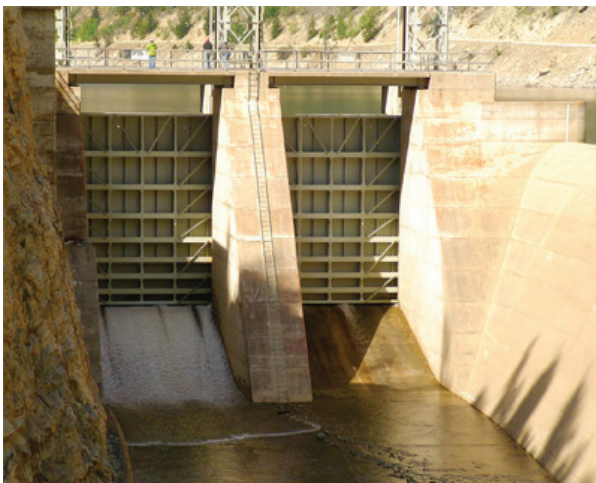
Figure 6.14: Vertical Lift Wheel Gate
